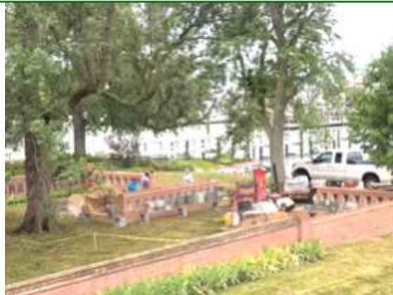
Columbarium Work In Progress
